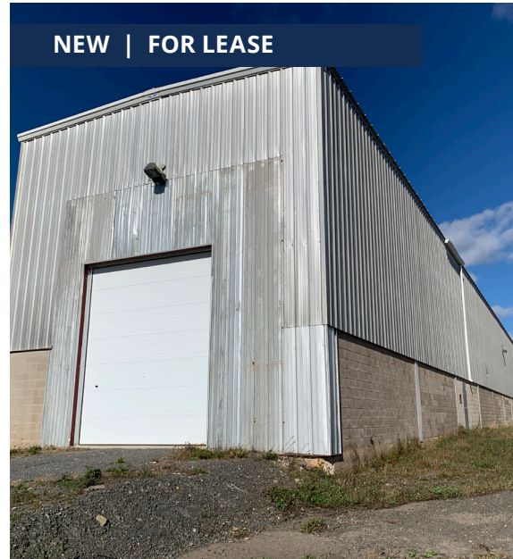
819 ROYAL ROAD, BUILDING H2, FREDERICTON
